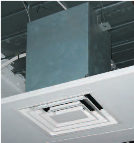
Typical Installation with Side Entry Plenum
